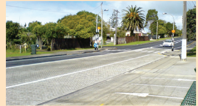
The 200 m 2 section of permeable pavement on Birkdale Road on the North Shore.
